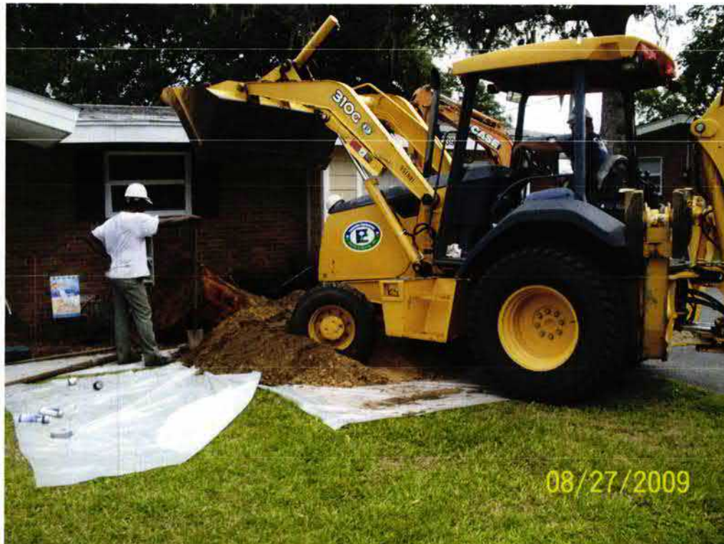
Picture 2: UST 1239Dove being removed.
